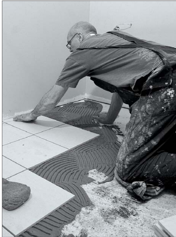
John Seman lays tile for the bathroom floor March, 5 2010 at the future school site for the St. Clair journalism program.
